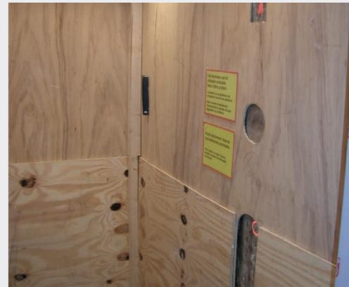
**KONE Construction Time Use elevators** are the final elevator equipped with protective materials so they can be used during construction. This means they operate at the same speed and load capacity as designed to move people and materials quickly and safely around the site. Before handover, the lift interiors and signalisation are installed and protective items removed to reveal the new elevator.
