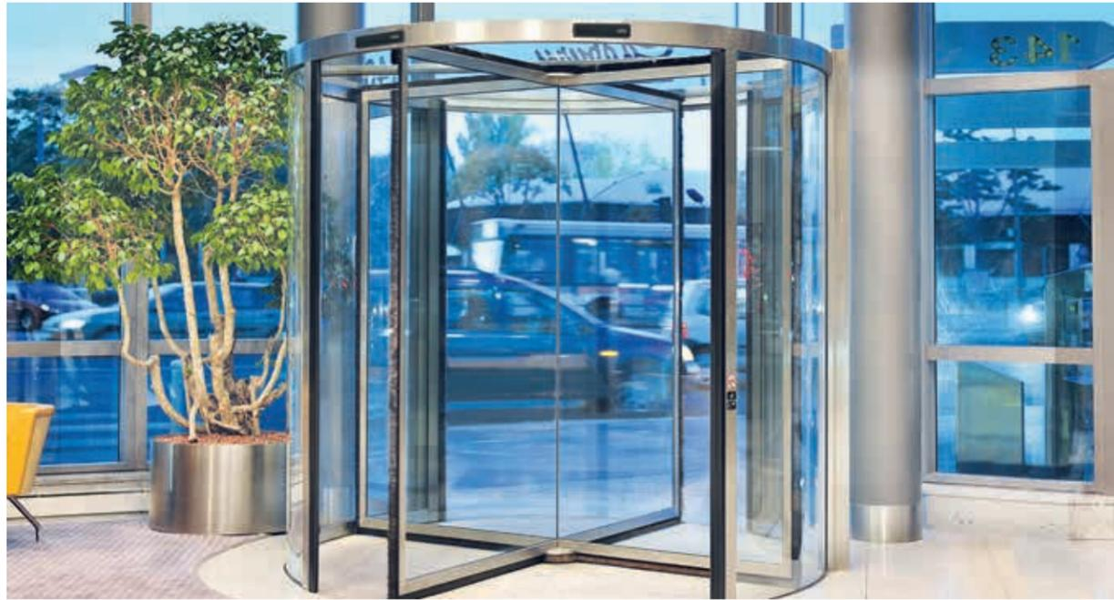
A typical office building features a wide range of different door types, including revolving, sliding, swing, and gliding doors. Lobbies may also include turnstile solutions to improve people flow, enable secure access control, and provide clear guidance for building users.
